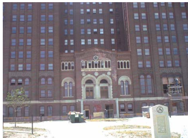
Project: Livestock Exchange Apartments Customer: Tufly Drywall
